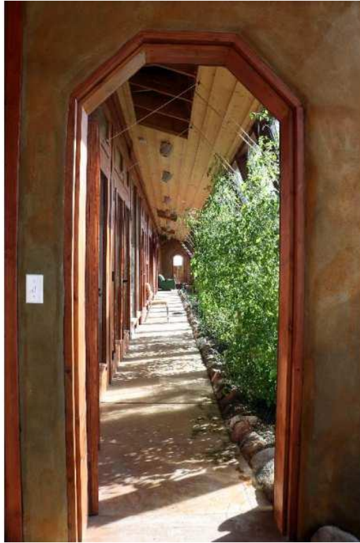
Looking into the Kinney earthship's long greenhouse, which serves as a main hallway and air barrier between the living space and the outdoors. It also produces vegetables year round. Christina Ryan / Calgary Herald
