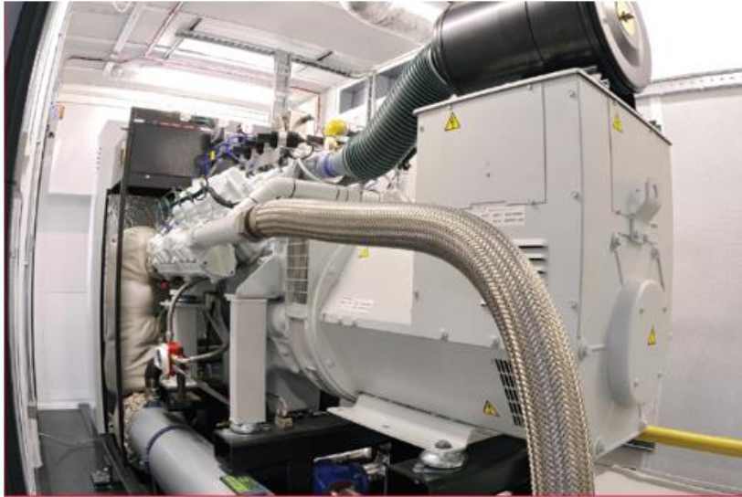
This is a picture of a reciprocating engine based CHP (the most efficient option), shown within its noise attenuated, anti-vibration enclosure surrounding it. Source: Ener-G
